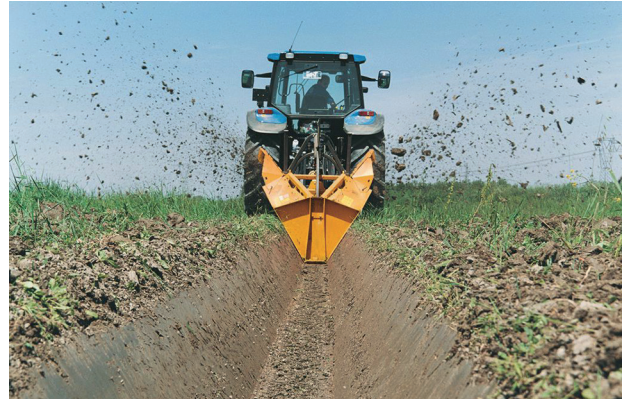
Construction of melioration facilities, closed horizontal drainage and collector
