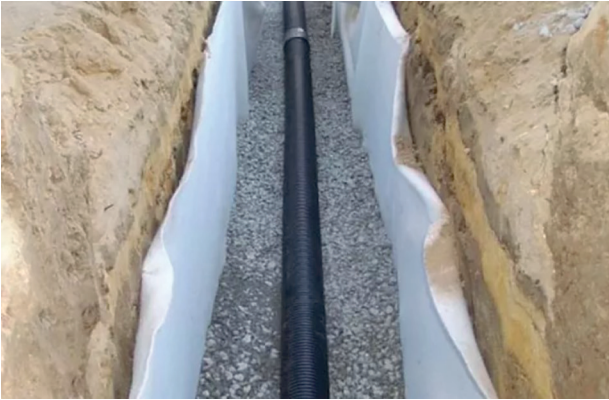
Construction of melioration facilities, closed horizontal drainage and collector
